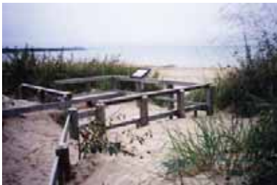
Sand mobilization through the dune blowout has led to extensive accumulations on the viewing platform and adjacent trails
