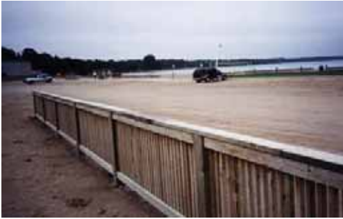
Permanent sand fencing on Port Elgin Beach parking area is designed to aid in trapping sand as well as assist the flow of traffic and parking.
