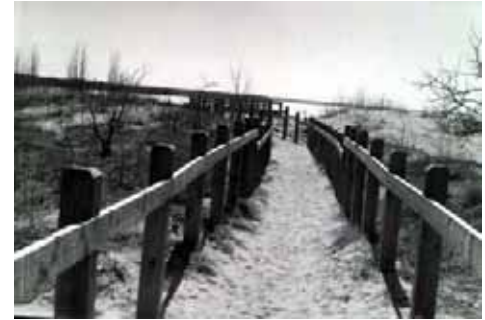
Post-and-rail pathways to control access through the dunes at Southampton.
