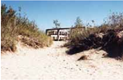
Breach in the foredune exposing the viewing platform to sand burial.
