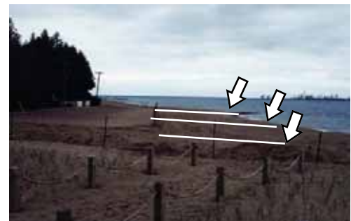
At locations like Wellington St., placement of fences perpendicular to southwest wind
