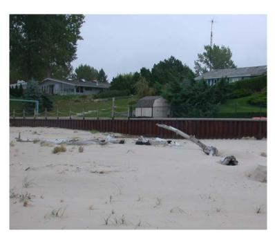
Seawall built in this dune area isolates the sand behind the wall from the active beach. In this example, the owner has not only built a seawall, but has built a cottage directly on the dune.
